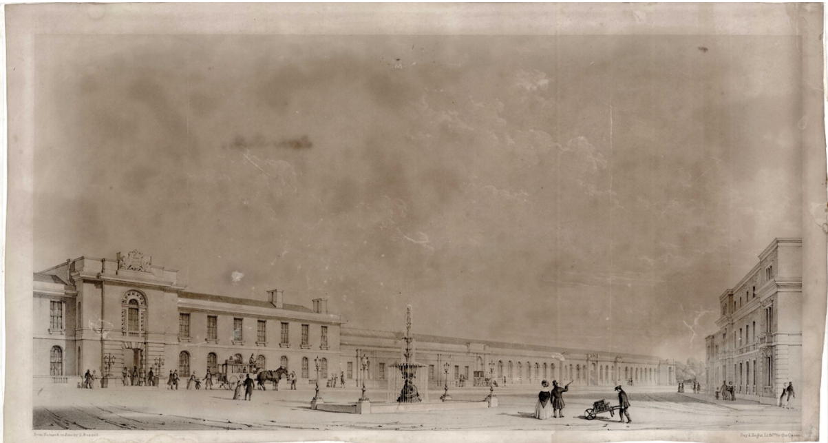
Lithograph of the 1840 front of Derby Station, designed by North Midland Railway architect, Francis Thompson, and drawn from real life by Samuel Russell. Courtesy of Midland Railway Study Centre
